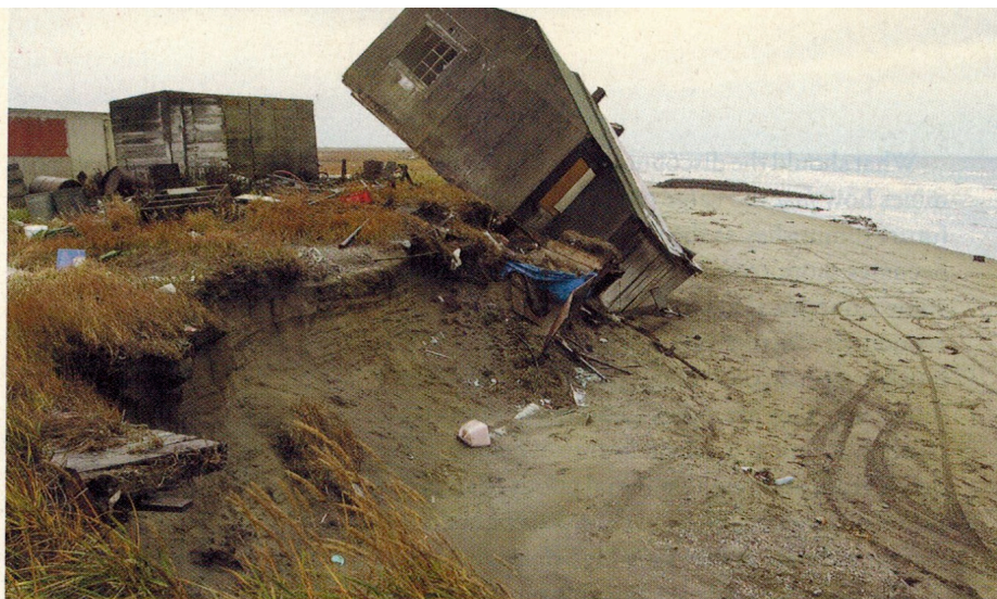
DEVASTATING COASTAL EROSION in the Alaskan village of Shishmaref, caused by the loss of permafrost and storm-buffering sea ice in a rapidly warming climate, is forcing the villagers to abandon their island homes and relocate to the mainland.
